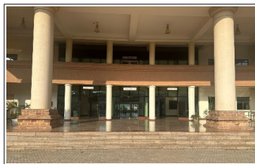
Image 3: Pillars base made out of laterite blocks in NISER Bhubaneswar
